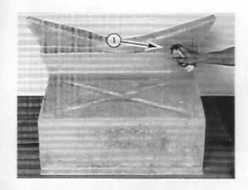
Cut insulation 30" long X roll width.
