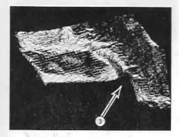
3 Fill voids with insulation trimmings.
