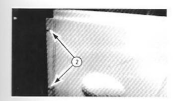
2 Insert two painted carriage bolts and secure with fender washer, lock washer and nut.
