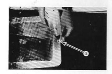
4) Align the previously drawn lines on the bottom of seat with seat box. Using hinge as a guide, drill two 3/16" holes into seat bottom. Attach seat bottom to hinge with two 3/16" rivets.
