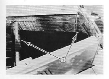
3 Place plywood floor in position, allowing studs to pass through the holes in the floor.
