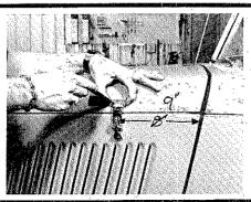
With a hacksaw blade or a grinder, remove any excess bolt protruding above the nut and paint the nuts black (excess bolt will scratch the side panels.)
