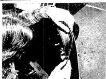
Install 1/8" x 3/8" weather strip around the perimeter of the front door edge.
