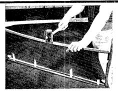
With your razor blade knife, carefully cut and remove the rubber to form neat 45° corners.
