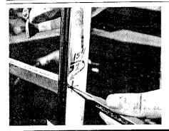
Measure in 15/32" and visually mark the correct vertical distance to install the frame connection screw. Drill a 13/64" hole perpendicular to the frame. Use your countersink bit to give a professional finish. Install the two screws and remove your binding wire. Install the rubber extrusion to the bottom frame member.
