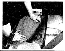
Drill  $\frac{1}{8}$ " holes around the perimeter of the box and into the top. Secure with wood screws.
